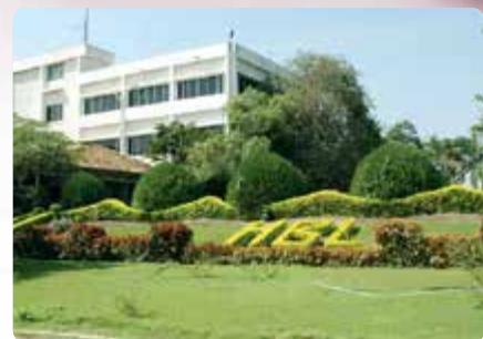
SHAMIRPET Hyderabad, Telangana Product line: Ni-Cd & Specialty batteries and power electronics
